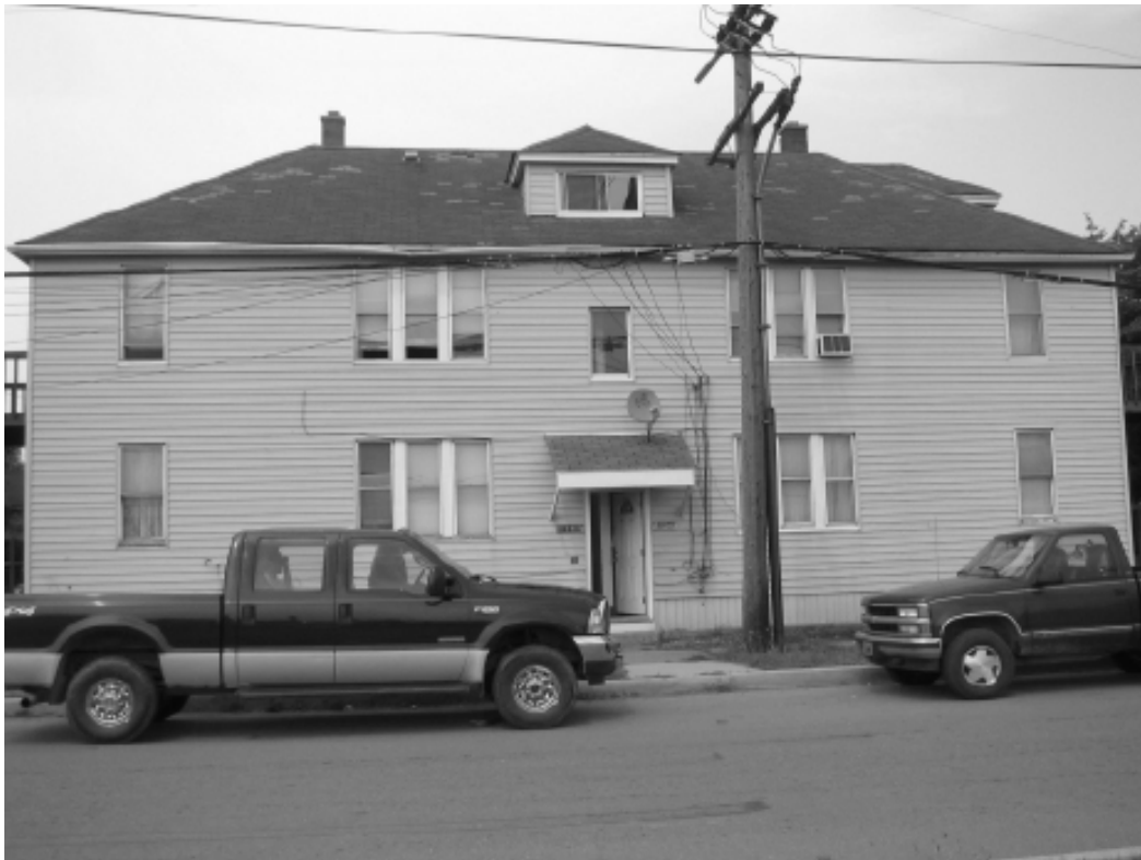
Figure DT-1 – Photograph of the residential structure in Detroit, Michigan
