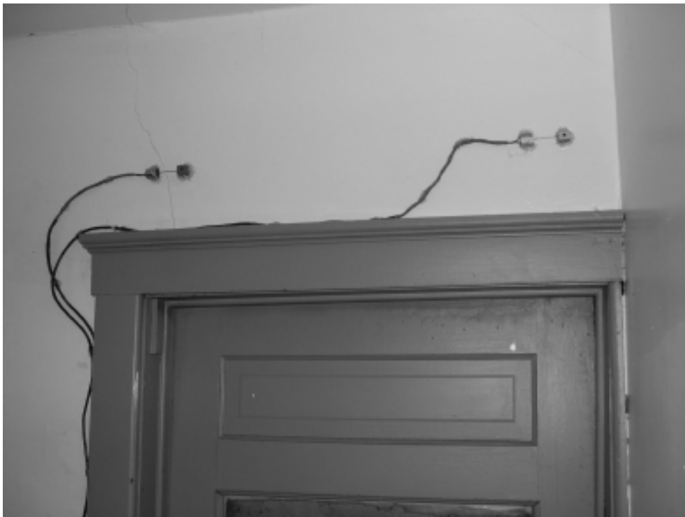
Figure DT-3 - Crack displacement sensor (left) and null sensor (right) installed in the stairwell above the back doorway to the upstairs apartment of the test structure.
